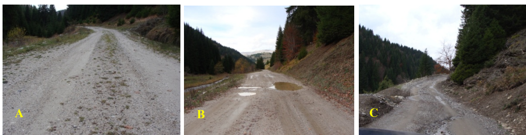
Figure 1. A – The good quality carriageway layer, B – The potholes, C – Bad carriageway layer (photo org. Halimić, 2012.)
